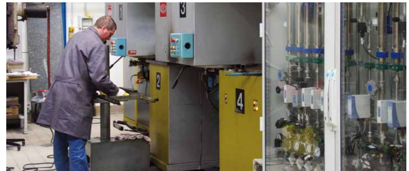
Fig. 1: Furnace for heat treatment using various processes at the foundation Institut für Werkstofftechnik (IWT) in Bremen
