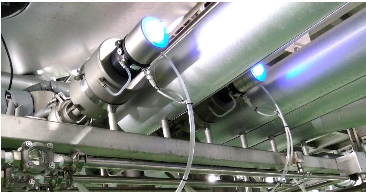
The Bürkert control heads Type 8691 (shown in the picture) and Type 8681 are highly adaptable, making it easy to combine them with various established process valves.
