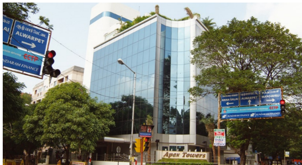
Bürkert Contromatic PVT Ltd, Chennai, India Apex Towers, 54 II Main Rd, R.A.Puram.
